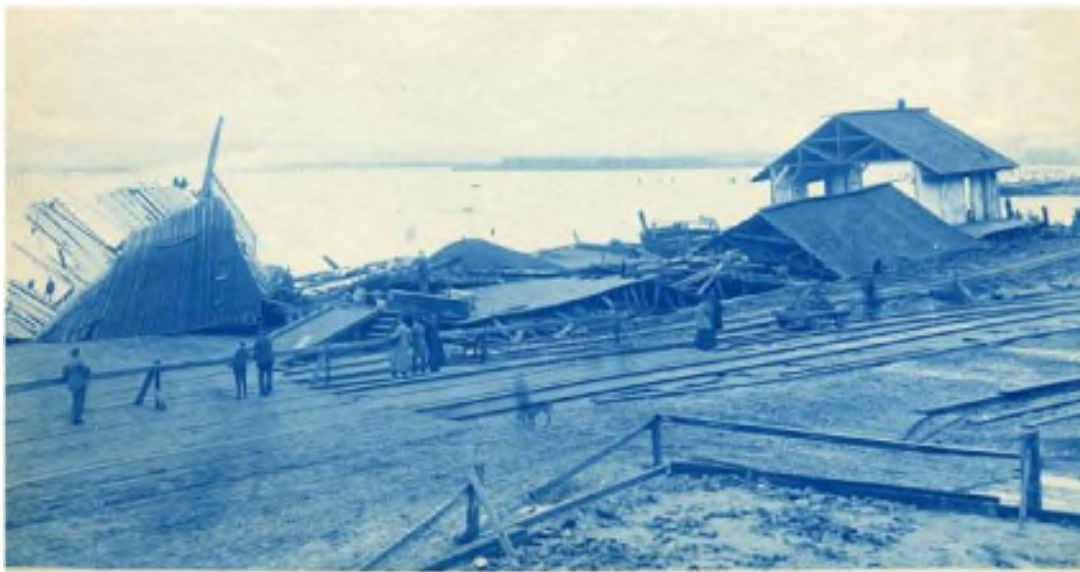
Figure 9. Damage in Tacoma from the 1894 Tsunami 14
