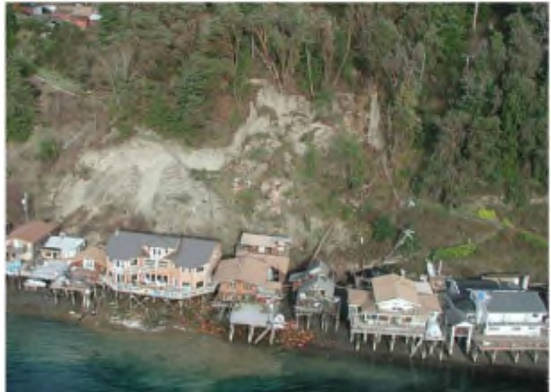
Figure 12. Salmon Beach, Tacoma, WA following Feb. 2001 Earthquake
