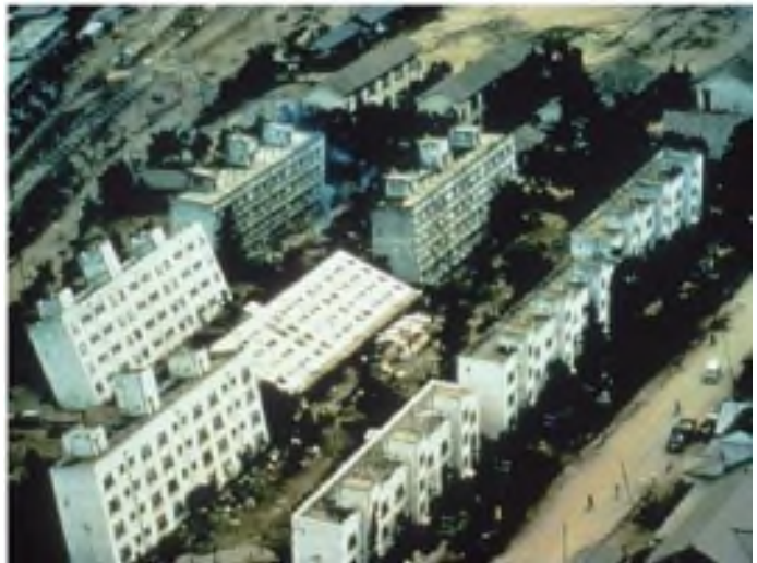
Figure 13. Liquefaction, Niigata Japan, 1964.
