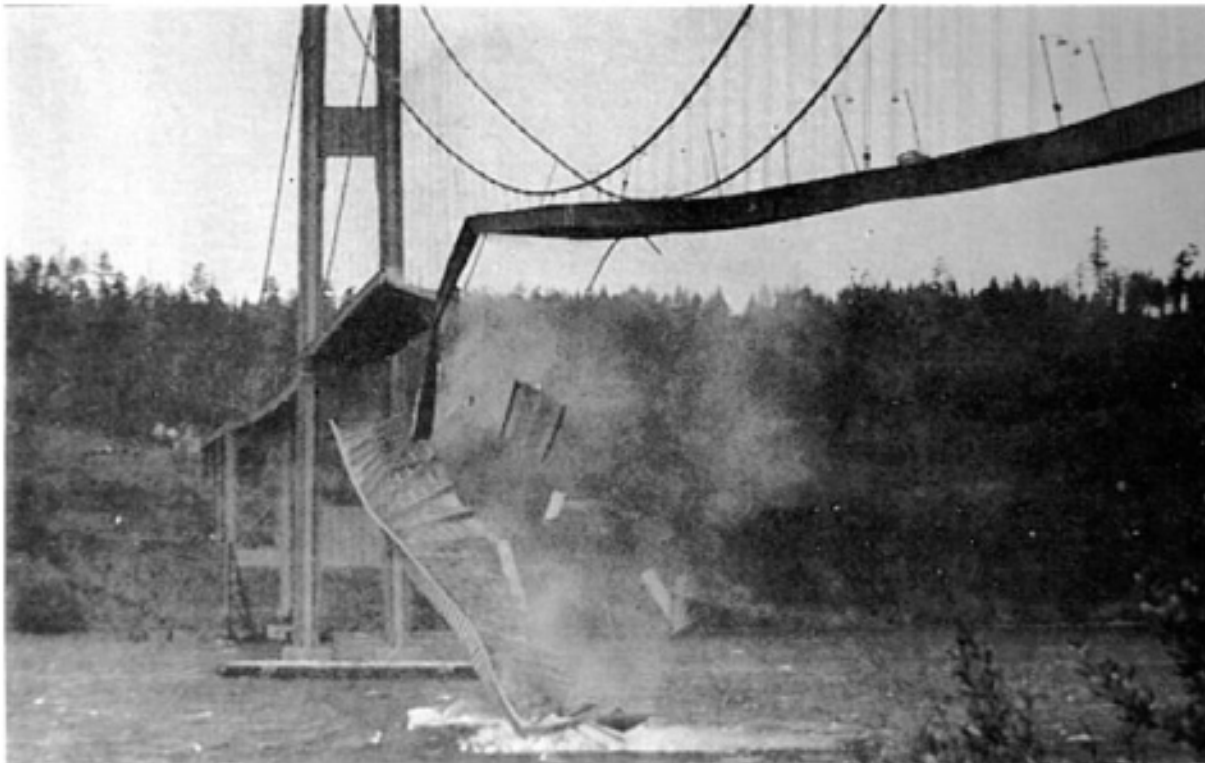
Figure 4. Tacoma Narrows Bridge, November 7, 1940 Windstorm 7
