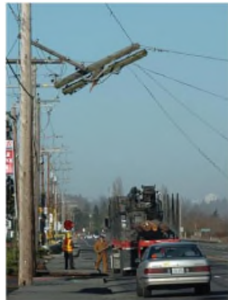
Figure 11. Impacts to Property and Infrastructure
