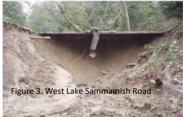
Figure 3. West Lake Sammamish Road Damaged after Landslide in January 2012
