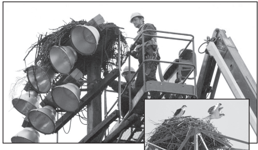
Contractors for Bellevue retrieve an osprey nest from the light pole.
