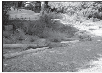
Plantings, gravel, logs and slope modification (left) can be an effective alternative to bulkheads (right).
