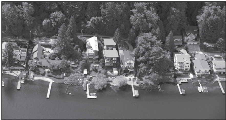
Docks and bulkheads dominate the Lake Sammamish shoreline.
