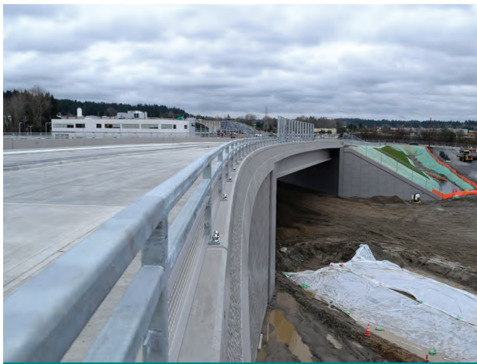
The first section of Northeast Spring Boulevard, with overpass for East Link, is complete.
